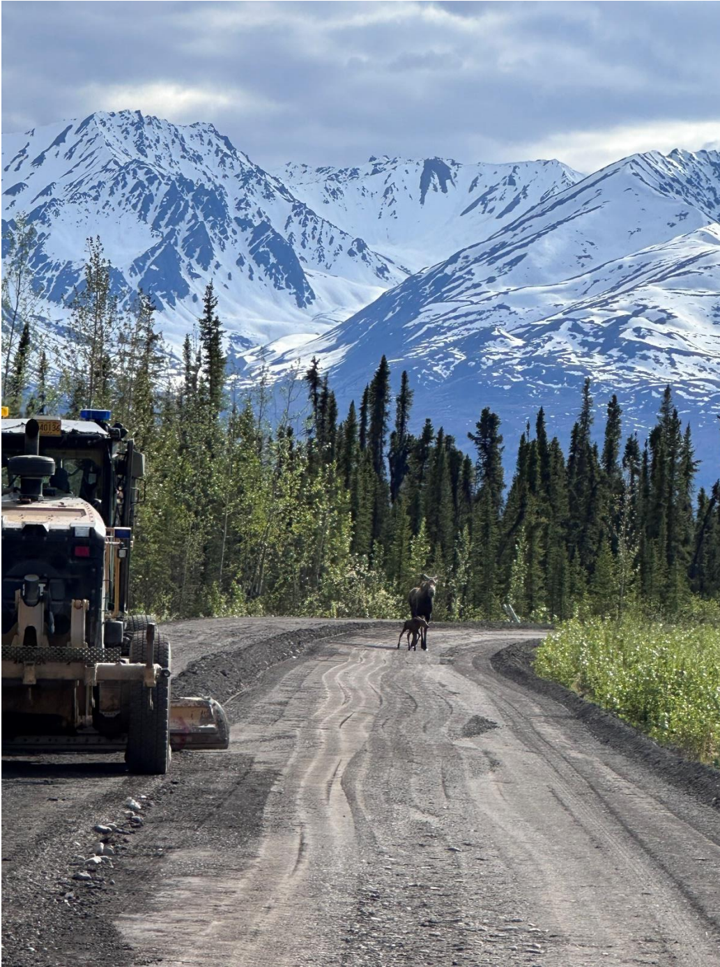
Figure 1. Spring blading at Mentasta Spur MP 5.
